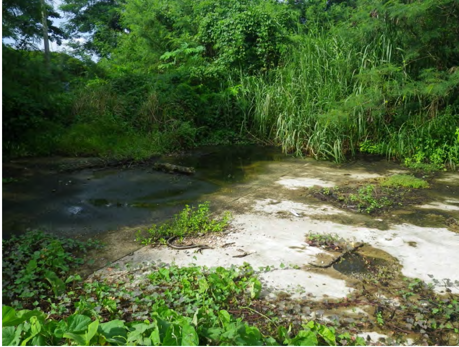
FIGURE 7-18. CONCRETE PAD, FEATURE 9.
