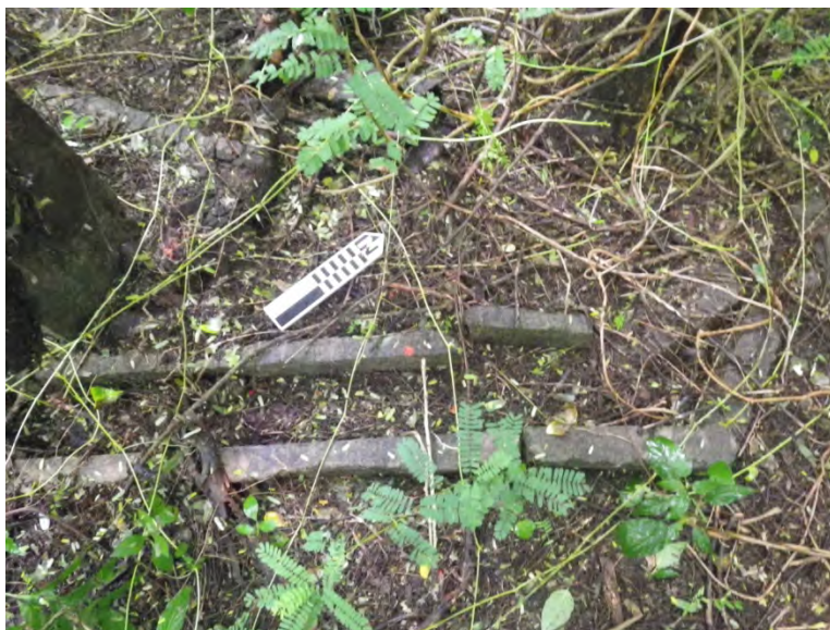
FIGURE 7-17. DRAINAGE LINE, FEATURE 8.
