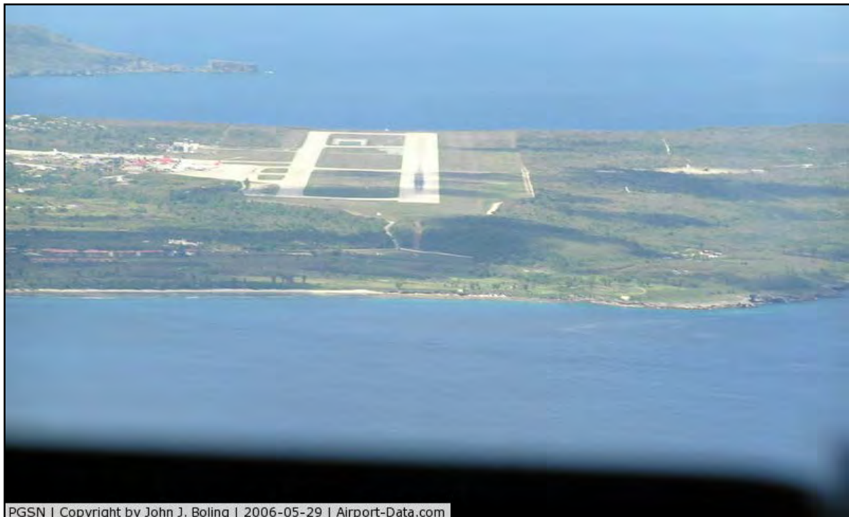
Figure 3.3-2. Aerial View of Saipan International Airport
