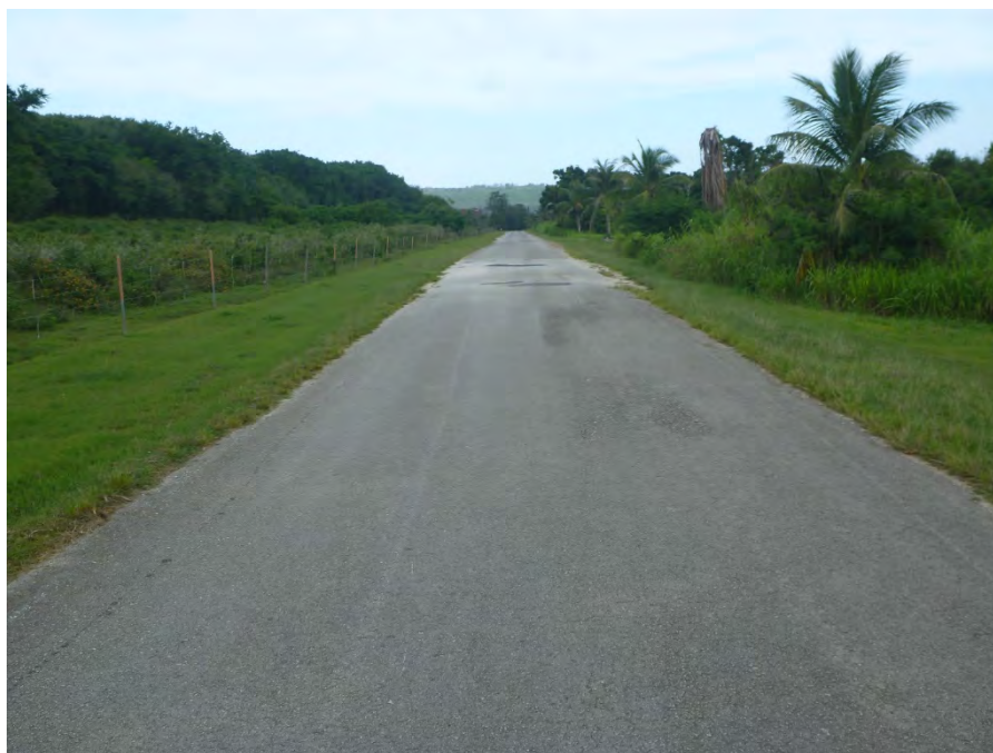
Photograph 14. View looking southeast on 42nd Street in proposed roadway improvement area outside an urban area.
