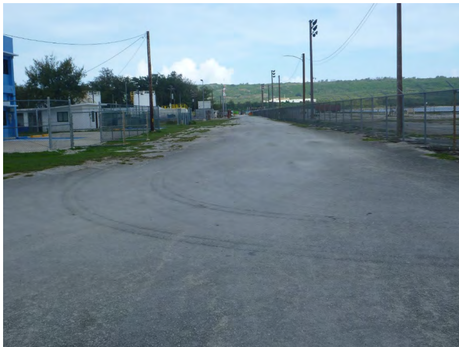
Photograph 8. Urban and Built Up vegetation near the seaport.
