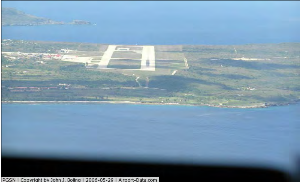
Figure 3.3-2. Aerial View of Saipan International Airport
